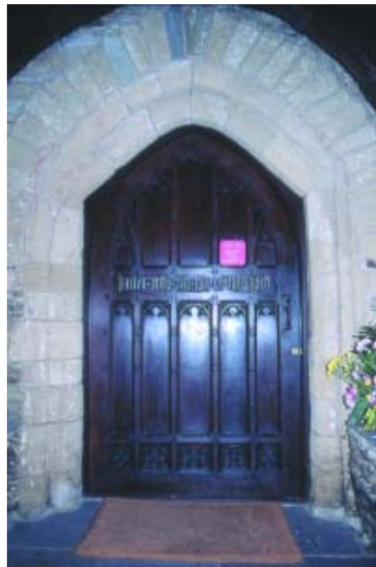
10. An arch built of Quaternary sandrock in St Carantoc's church at Crantock. A tower built of this sandrock in the 14th century fell down shortly after it was built, suggesting that there are structural limitations with this type of stone. (c. Colin Bristow)
