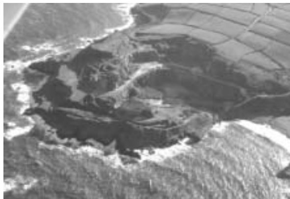
Figure 3: West of England Quarry, Porthoustock. This Gabbro quarry is typical of aggregates quarries in having few waste dumps and the interior is relatively formless. Few structural remains survive here except parts of the jetties. Prograded beach at Porthoustock shows on the right. (c. Historic Environment Service, Cornwall County Council)
