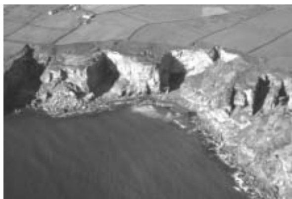
Figure 2: Bagalow, south of Tintagel. Each of the inlets in the cliffs are coastal slate quarries where the cliff faces have been formed by workings. Horse whims (winding capstans) and dressing sites lie on top of the cliffs. The quarries from left to right are Dria, Bagalow, Caroline, and Lanterdan. (c. Historic Environment Service, Cornwall County Council)
