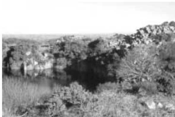
Figure 2 Flooded former dimension stone quarry at Higher Trolvis, near Longdowns. Note the waste tip on the right composed of large flawed blocks of granite. There is around 1.5 km 2 of land affected by granite quarrying in the Carnmenellis granite. (c. Colin Bristow)
