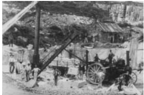
Figure 4 Polkanuggo quarry, near Mabe, towards the end of the nineteenth century. A traction engine is loading blocks of granite onto a wagon. (c. Royal Institution of Cornwall)
