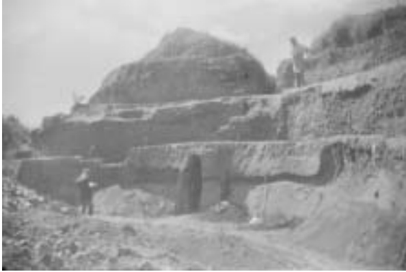
Figure 8 St Erth sand pits in about 1910. These sands and clays were used as moulding sands for casting iron and the clays were later used by Bernard Leach for his pottery. They have yielded a rich fossil fauna and flora which provides a valuable insight into climatic conditions just before the onset of the ice ages. (c. Royal Institution of Cornwall)
