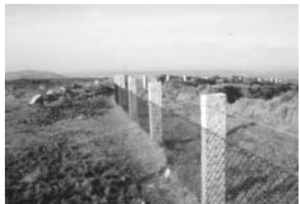
Figure 4: Granite fence posts between Holman's quarry and the public bridleway (c. Kerrier District Council)
