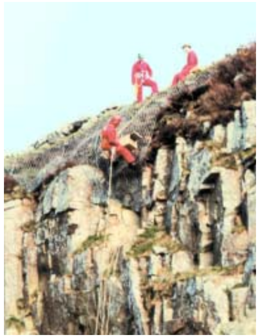
36. Installation of Kestrel's nest box, Holman's Quarry (c. Kerrier District Council)
