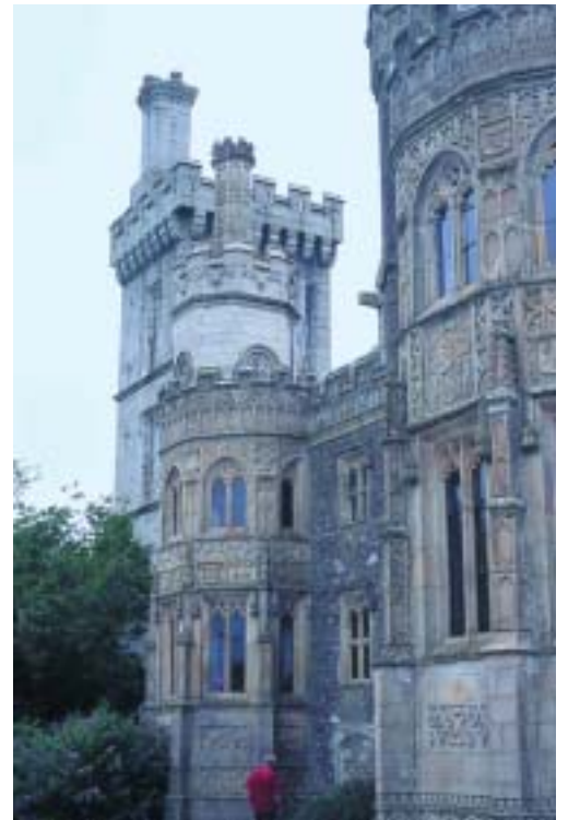
4. The exterior of Place, Fowey, faced with Pentewan Stone. Much of the stone was renewed in the early 19th century by Joseph Treffry, the famous mid-Cornwall quarrymaster, who lived at Place. The most likely source for this stone was a quarry inland from Pentewan village (SX 022479). (c. Colin Bristow)
